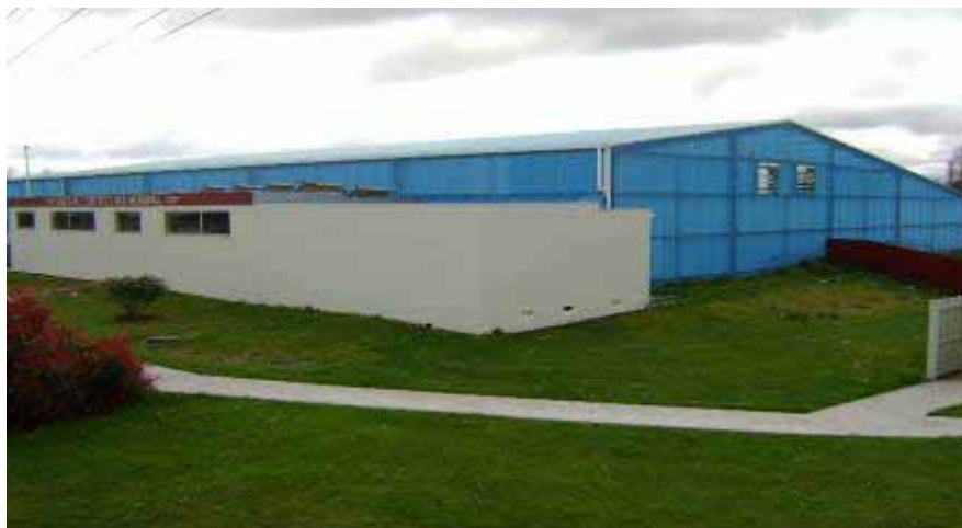
Raetihi Swimming Pool Complex – Parapara Road, Raetihi
