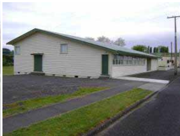
Manunui Memorial Hall – Council manages
