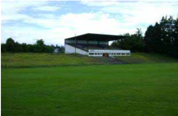
Taumarunui Domain Grandstand Domain, Morero Terrace, Taumarunui
