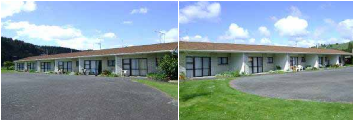
Taupo Road, Taumarunui Older Persons Housing Units
