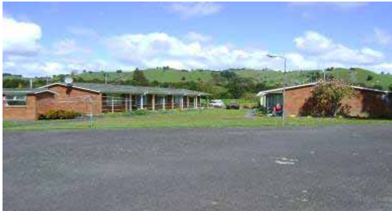
Taupo Road, Taumarunui Older Persons Housing Units 1-10
