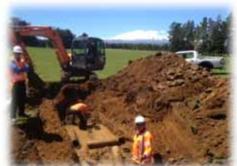
National Park reservoir roof replacement
