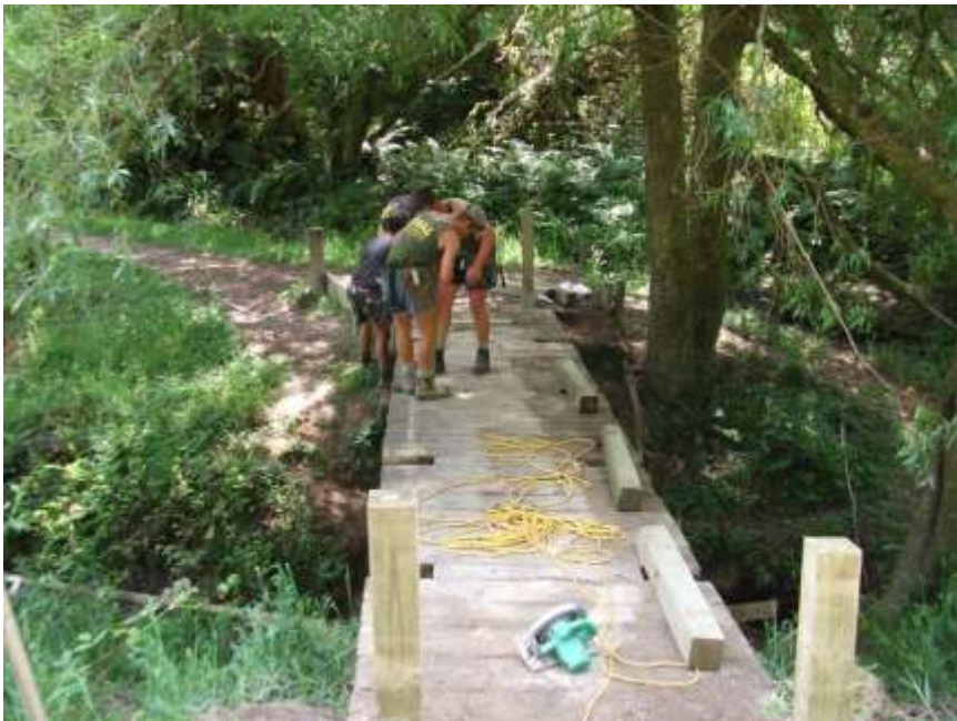
Roslyn Street Walk Bridge Upgrade
