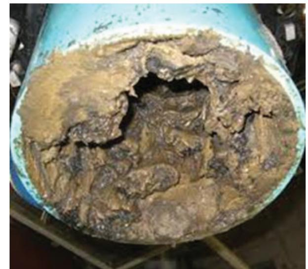
The sewer was almost completely clogged with over 15 tonnes of fat which had reduced the sewer to just five per cent of its normal capacity. The blockage was discovered after local residents complained of being unable to flush their toilets.
