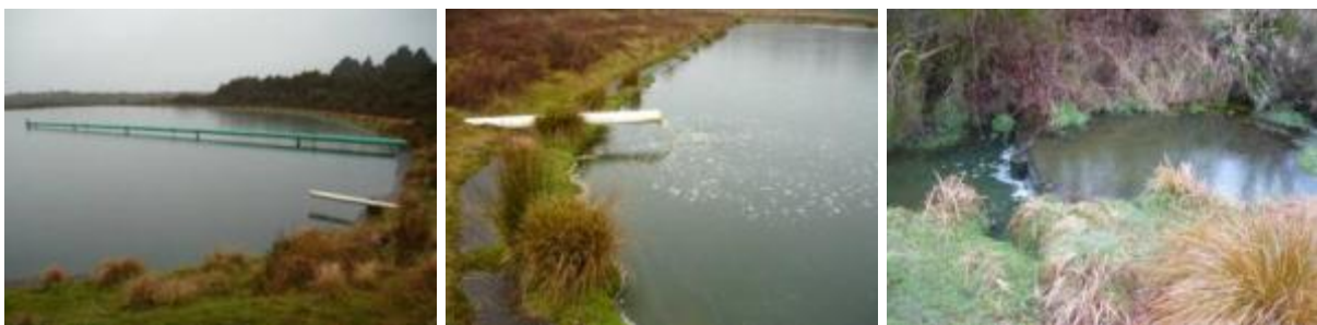
Primary oxidation lagoon (left), secondary oxidation lagoon (middle), First discharge weir (right)
