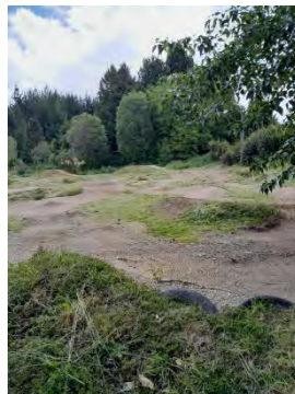
Major renovations, Ohakune Pump track
