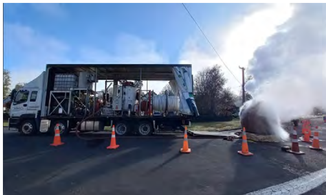
Relining works at North Street, Taumarunui
