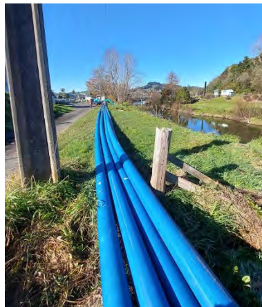
New watermain pipes laid out ready for installation
