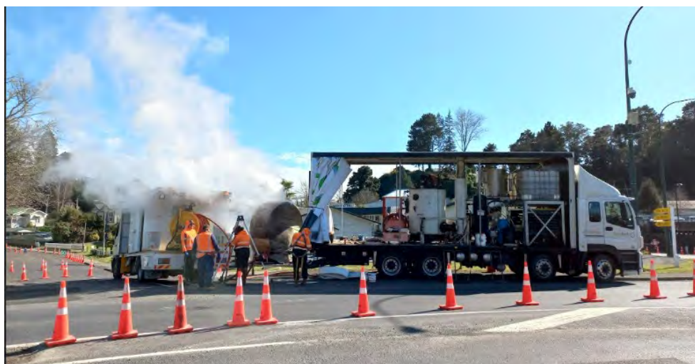
Relining works at the Ongarue Bridge, Kururau Rd intersection, Taumarunui
