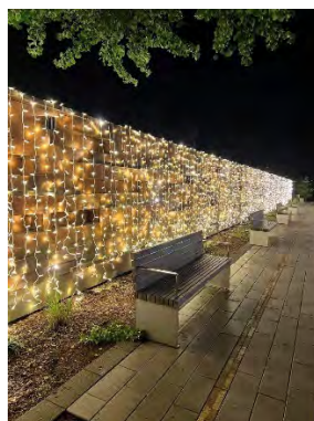
Christmas lighting & power installation
