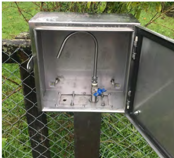
New water sample collection points
