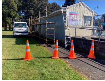
Taumarunui Pool Office Roof
