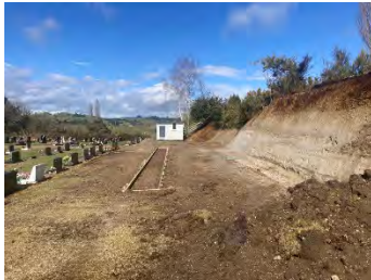
Manunui ashes Berm & Cemetery Wall preparations
