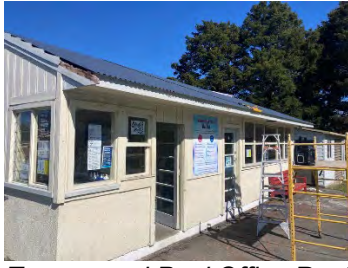
Taumarunui Pool Office Roof
