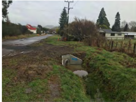
Culvert replacement – Plunket Street
