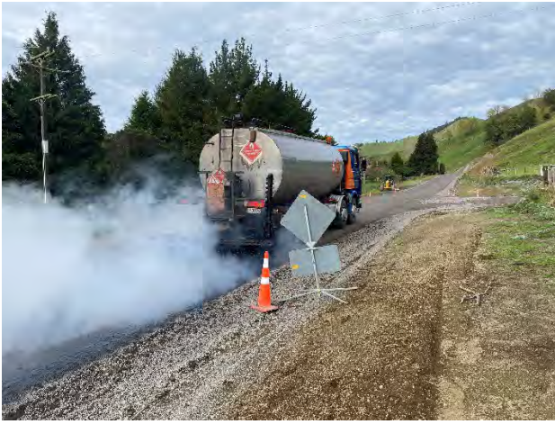
Sealing Ruatiti Road
