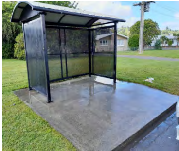
Bus shelter renovations District wide
