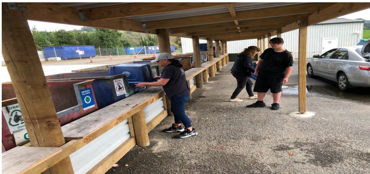
Taumarunui Refuse Facility under construction.
