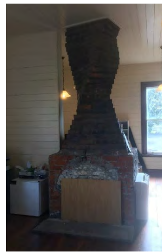
Internal Spiral Chimney (3) in ex-Visit Ruapehu Rooms
