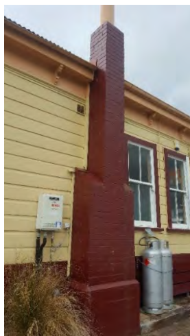
External Chimney (2) in shop end of building
