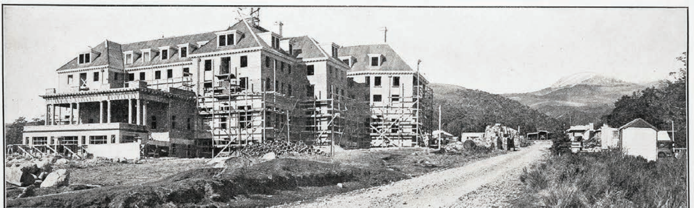
THE NEW ACCOMMODATION HOUSE AT TONGARIRO NATIONAL PARK, NORTH ISLAND, RAPIDLY NEARING COMPLETION. A recent photograph of Chateau Tongariro showing the progress made in its construction. In the distance Mount Ruapehu can be seen on the right of the photograph. —Staff Photographer.
