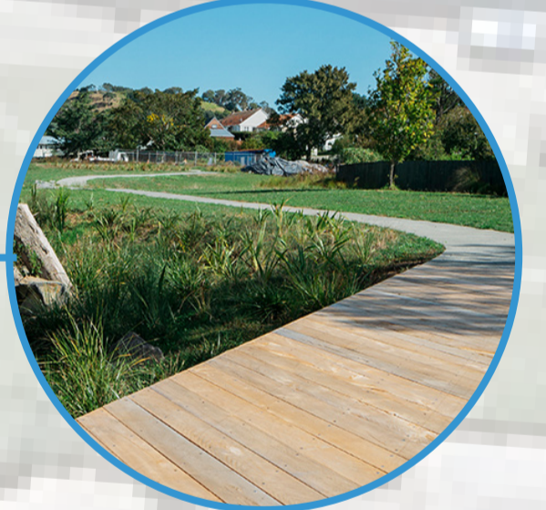
BRIDGE WITH DECKING / PLATFORM AND STEPS TO LOWER TERRACE
