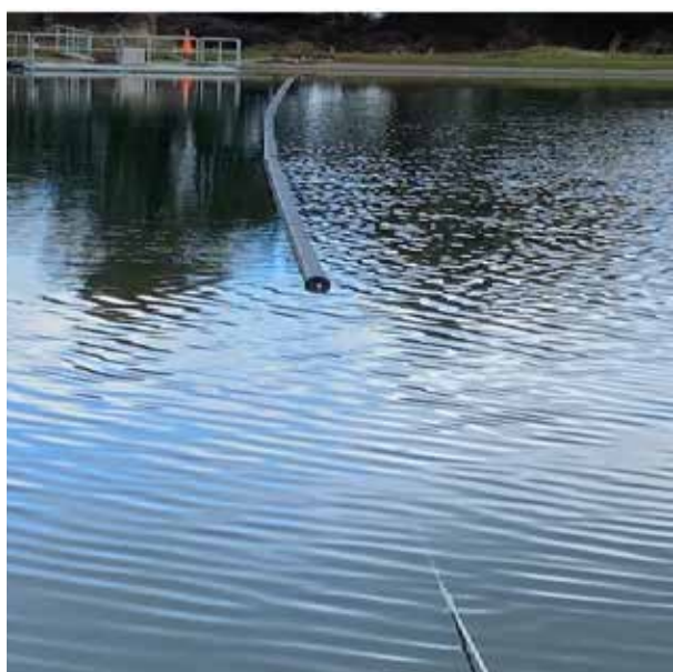
Ohakune WWTP – New baffle curtains installed.
