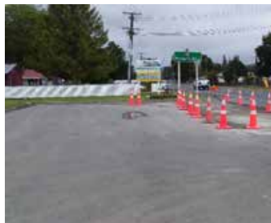
Raetihi Pool parking repairs.
