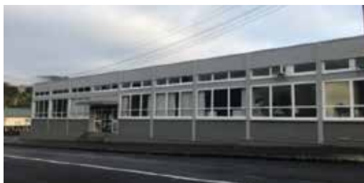
Miriama Community Centre repainted.
