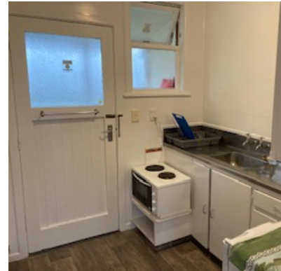
Painted kitchen, Rochfort Flats, Taumarunui.
