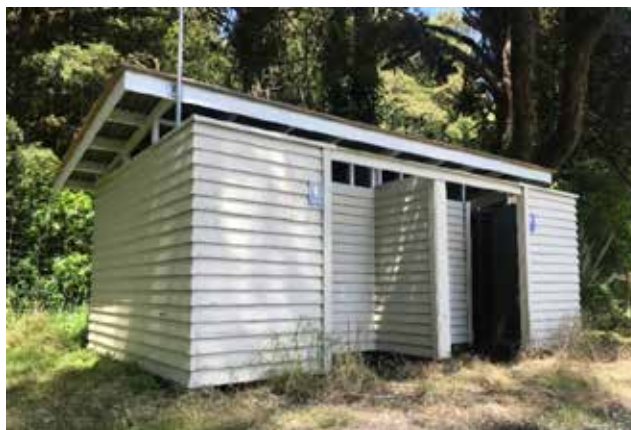
Manunui Reserve toilets painted.
