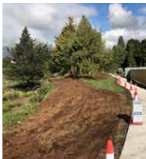
Raetihi Pool fence renewed and vegetation cleared.
