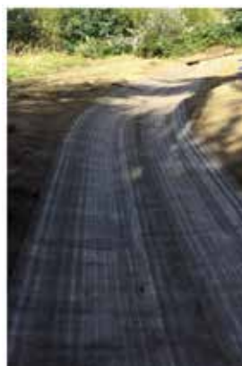
Pipiriki Stormwater - reformed swale drain.
