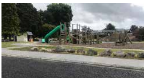
Taumarunui Domain Playground new carpark and footpath.
