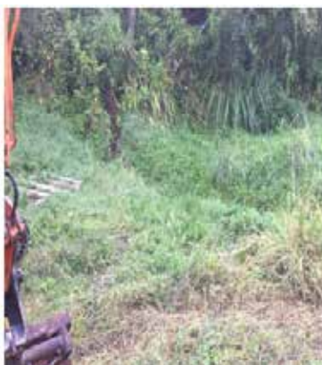
Pipiriki Stormwater – scoured stormwater drain.
