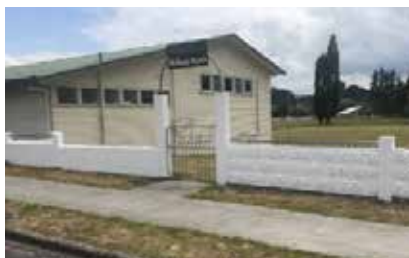
Manunui Hall fence painted.
