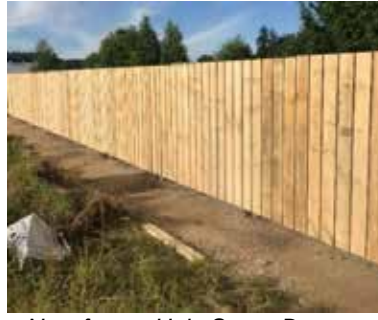
New fence, Huia Street Depot, Taumarunui.
