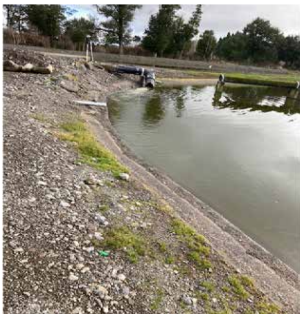
Ohakune WWTP – New discharge point at oxidation pond.
