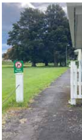
Restored fence alongside Taumarunui Pool.
