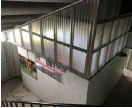
New clearlite panels, KCE Jubilee Grandstand, Taumarunui.
