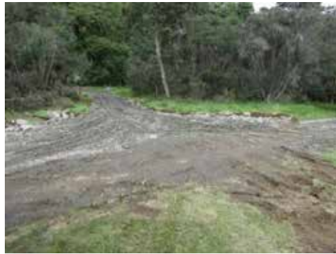
Gravel work on intersection of roads, Ruatiti Domain.
