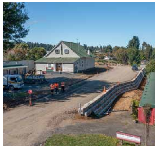
Rimu Street, Ohakune - seal extension under construction.
