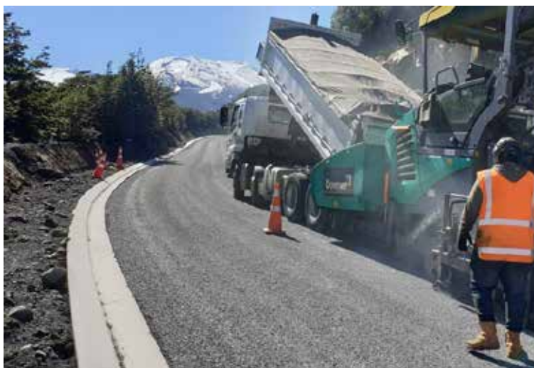
Asphalt being laid on Ohakune Mountain Road Hairpin at RP 13.50km.
