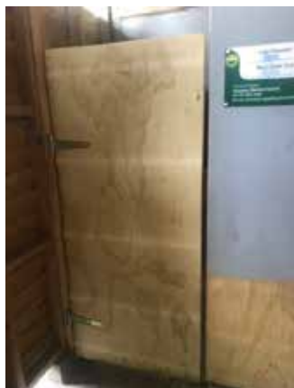
Manunui Reserve toilet doors improved.
