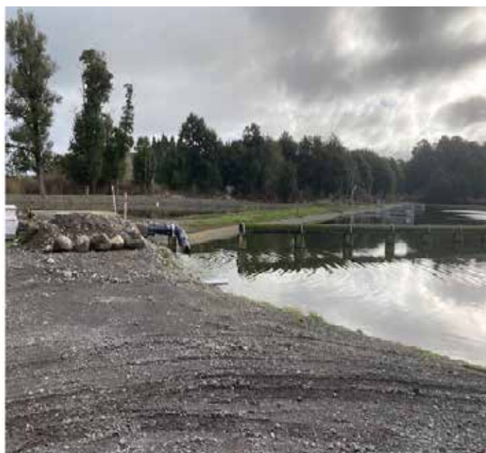
Ohakune WWTP – New discharge point at oxidation pond.
