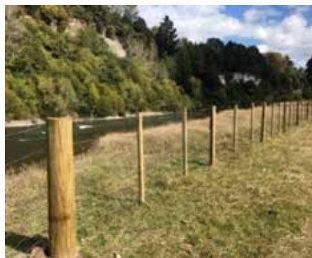
Sections of fencing completed along Whanganui River Accretion Land, Taumarunui.
