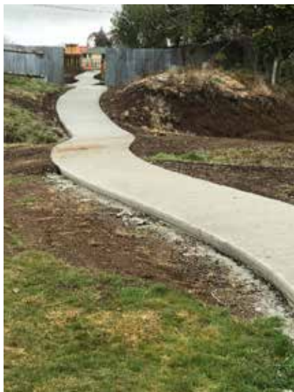
Makotuku Walkway, Raetihi accessible track extended.
