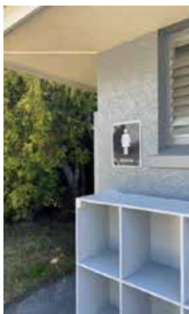
Taumarunui pool changing rooms after painting.
