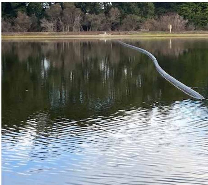
Ohakune WWTP – New baffle curtains installed.
