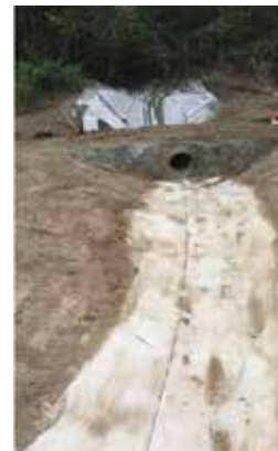
Pipiriki Stormwater – with concrete canvas.
