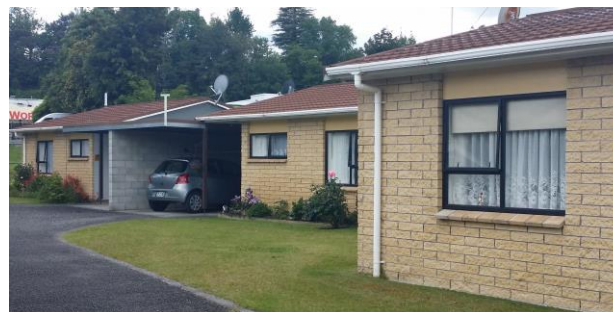
Miriama Street Flats, Miriama Street
