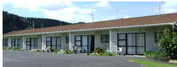
Rangimarie Flats, Taupo Road
