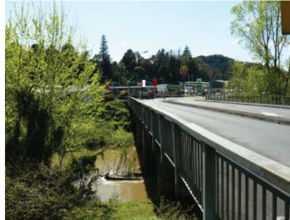
Kururau Road /Hakiaha St Bridge Orientation: North West
