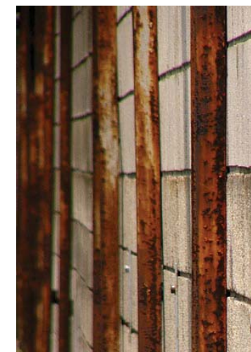
Steel and Concrete
