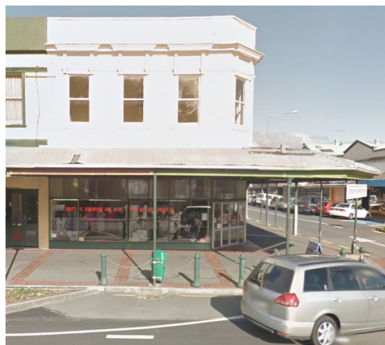
EXAMPLE 1: Corner verandah to Manuante St and Hakiha St works well to have pillars, and a profile that has a mild architectural rounded corner.
