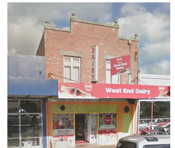
EXAMPLE 5: Vertical signage that is attached to the building and has historic value is to remain.
