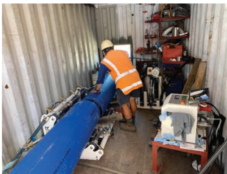
Welding new water mains for Golf Road prior to installation
