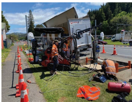
Relining of the Hakiaha Street sewage main
