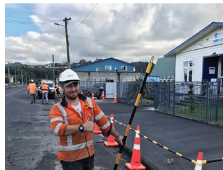
Footpath renewal on Huia Street
