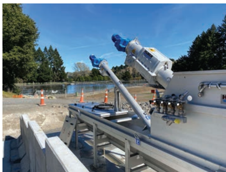
New screen technology being installed at Hikumutu Wastewater Treatment Plant
