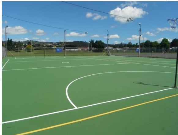
Netball Courts, Turaki Street, Taumarunui
