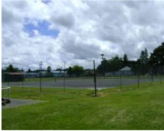
Tennis Courts, Parapara Road, State Highway 4, Raetihi
