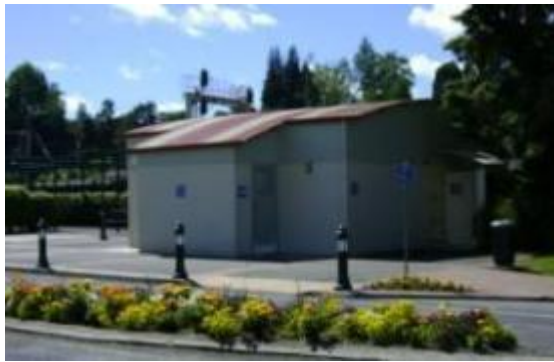
Hakiaha Street, State Highway 4, Taumarunui
