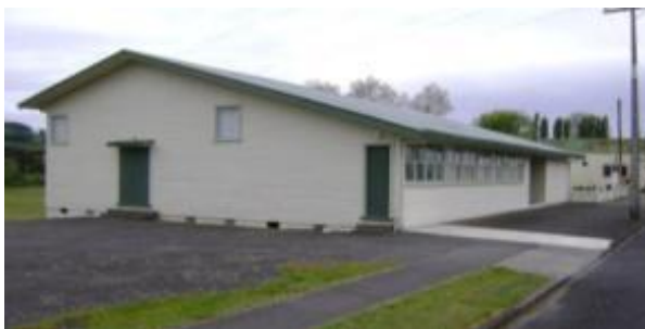
Manunui Memorial Hall (Managed by Council)
