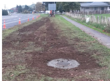
State Highway 4, Raetihi New Stormwater Line
