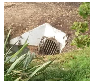
Installing a New Wing Wall, Taumarunui
