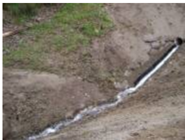
Improving Outfall of Stormwater
