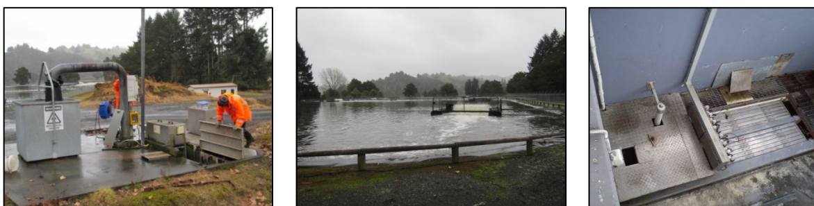
Figure 12: Treatment plant examples
