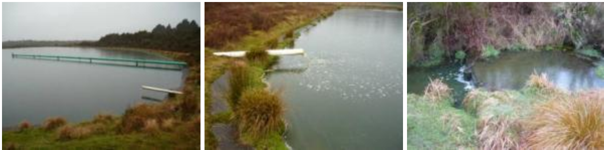
Primary oxidation lagoon (left), secondary oxidation lagoon (middle), First discharge weir (right)
