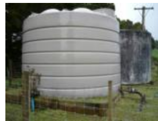
Sunshine Road Reservoir
