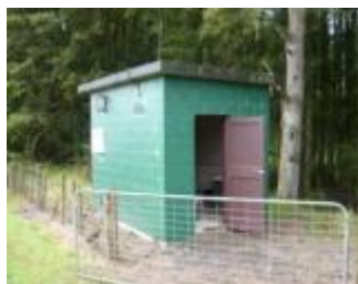
Manunui Booster WPS, Taumarunui
