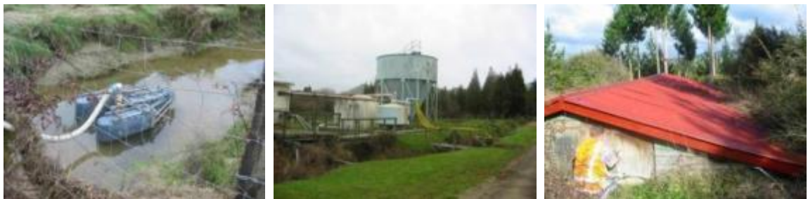
Mangaparare Stream intake (left), Ohura WTP (middle), reservoir (right)
