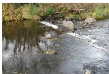
Raetihi WTP Intake Weir
