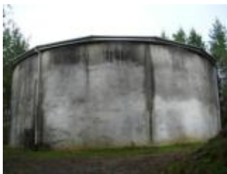
Matapuna Concrete Reservoir
