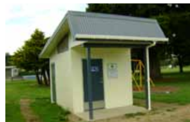
Taumarunui Domain Toilets
