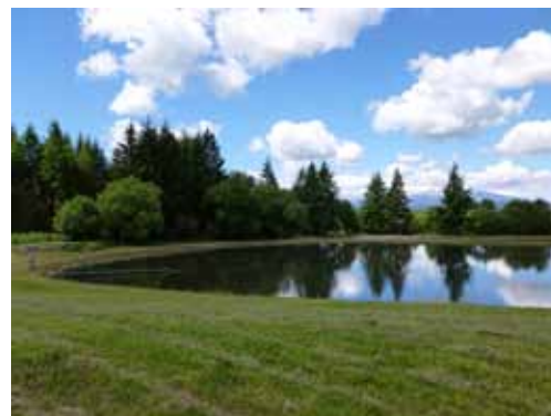
Ohakune Wastewater Treatment Ponds
