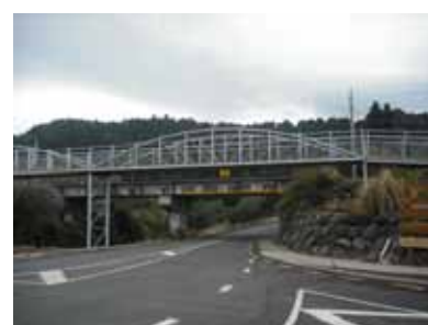
Pedestrian Bridge, Thames Street, Ohakune
